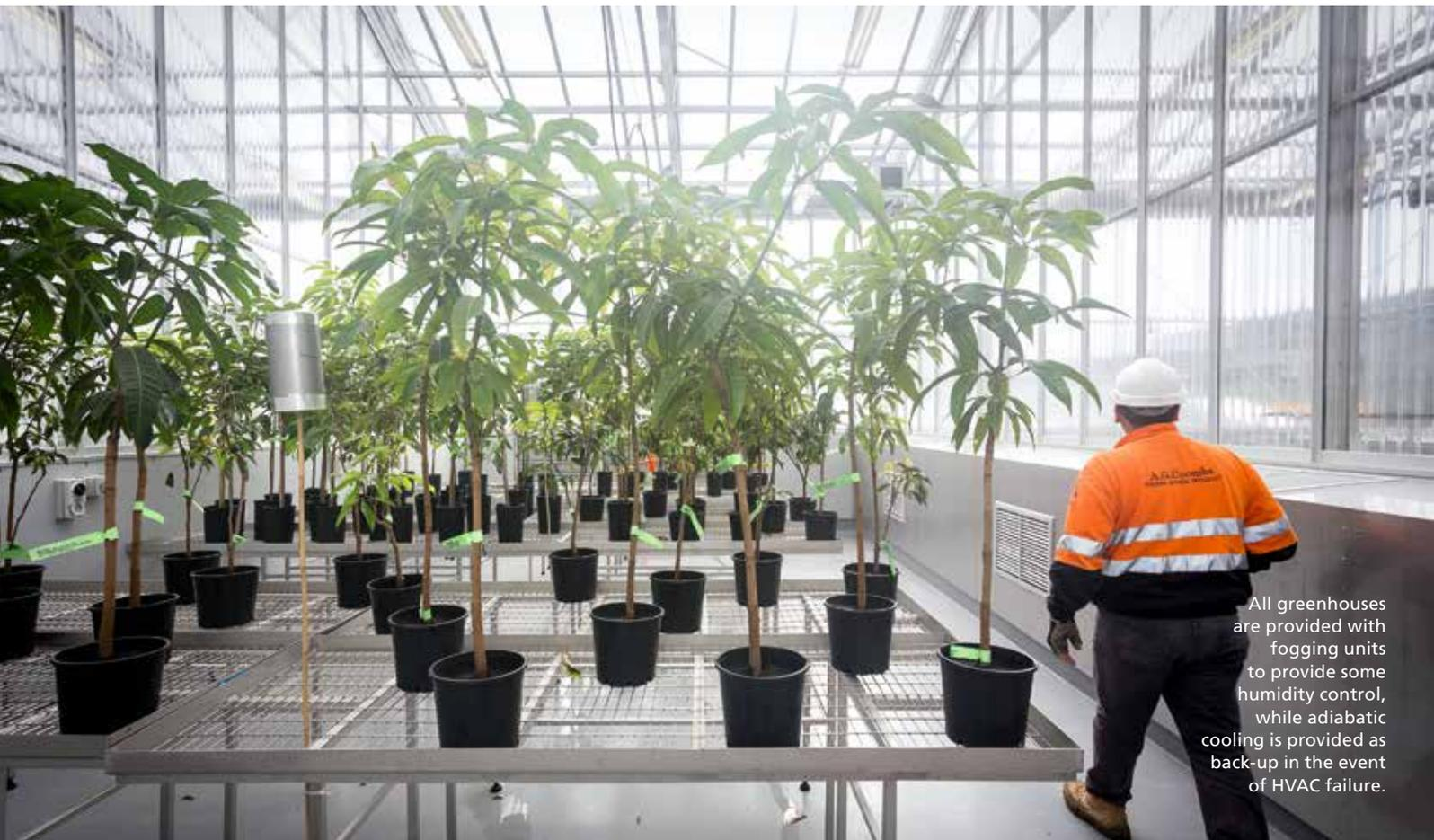
All greenhouses are provided with fogging units to provide some humidity control, while adiabatic cooling is provided as back-up in the event of HVAC failure.
