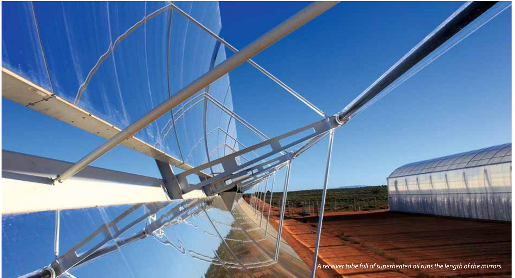
A receiver tube full of superheated oil runs the length of the mirrors.
