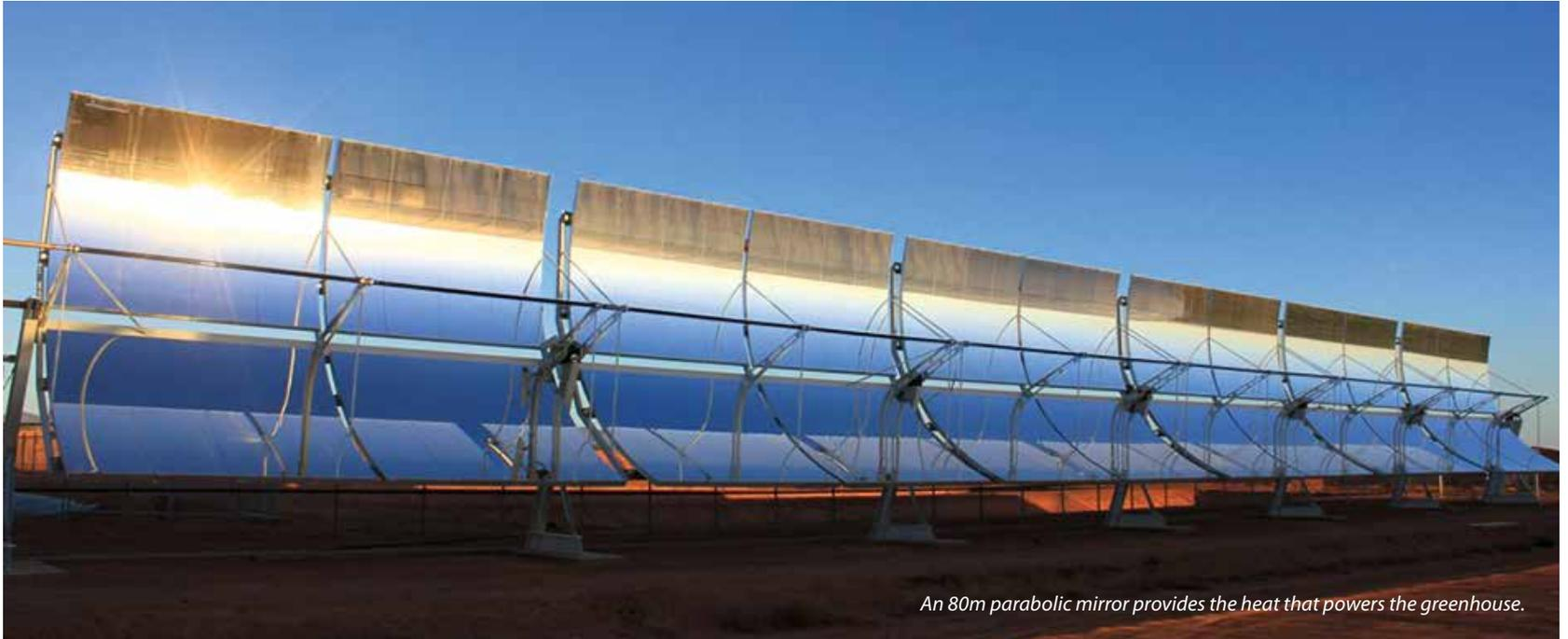
An 80m parabolic mirror provides the heat that powers the greenhouse.
