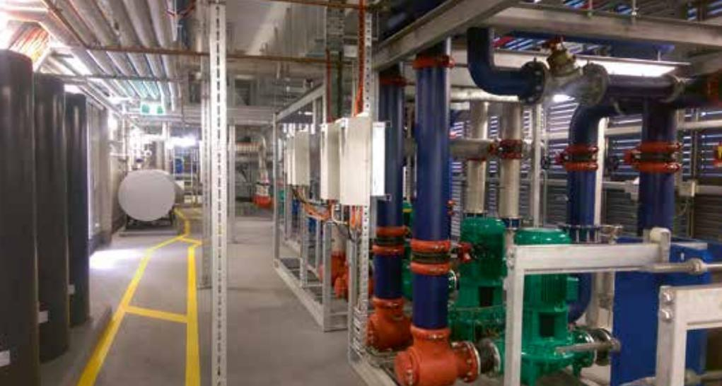
The use of pre-fabricated pump skids helped minimise the on-site installation times at 180 Brisbane. Image: A. Gattland, AE Smith.
