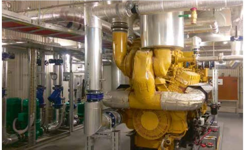
The trigeneration systems' 1MWe gas generator, located on level 33. Image: A. Gattland, AE Smith
