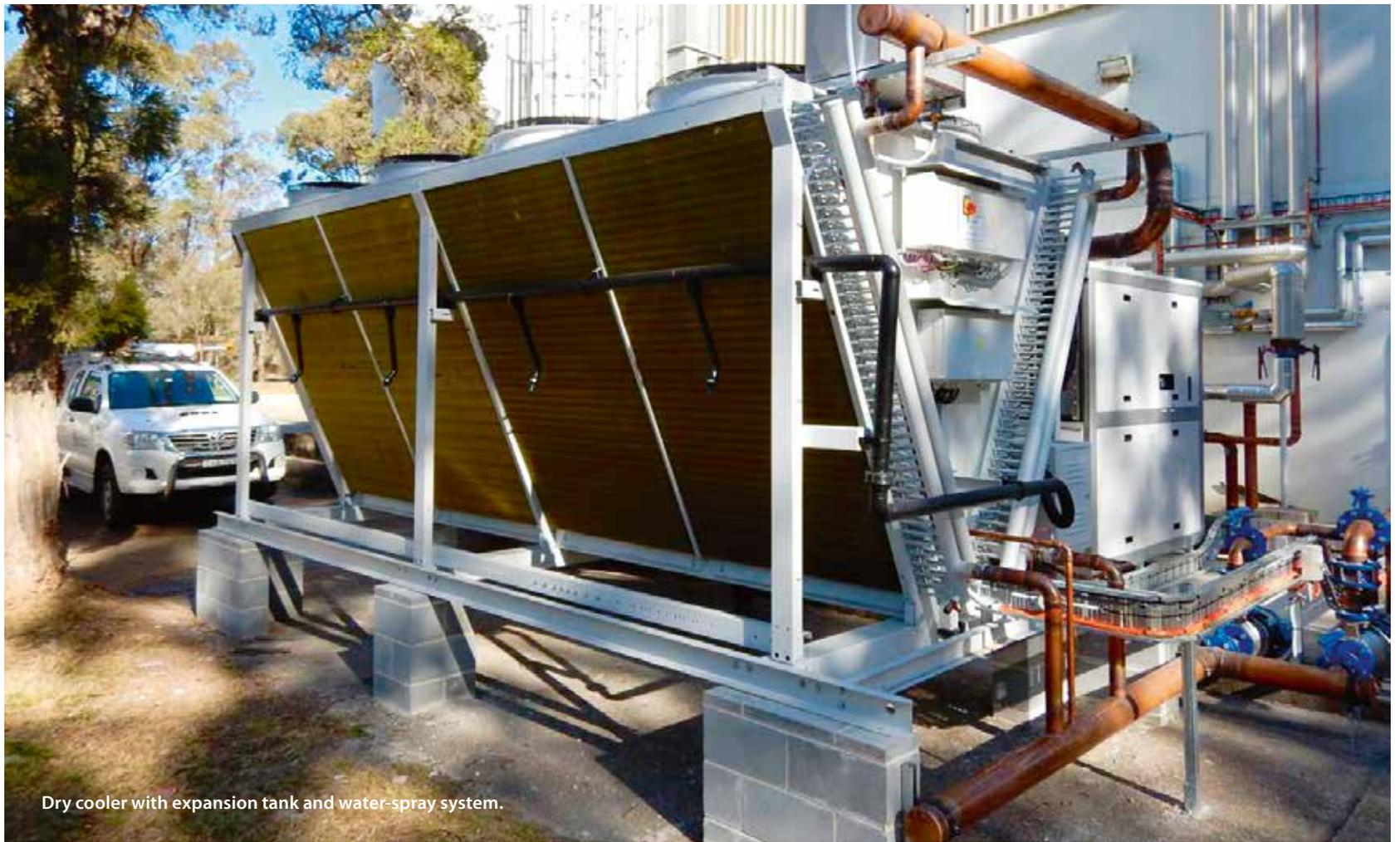
Dry cooler with expansion tank and water-spray system.
